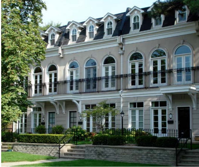
Low-rise building with articulated architectural features.
