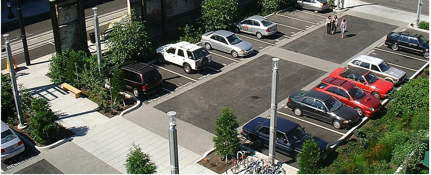
Surface parking lot that includes parking courts, plantings, lighting, and pedestrian walkways.
