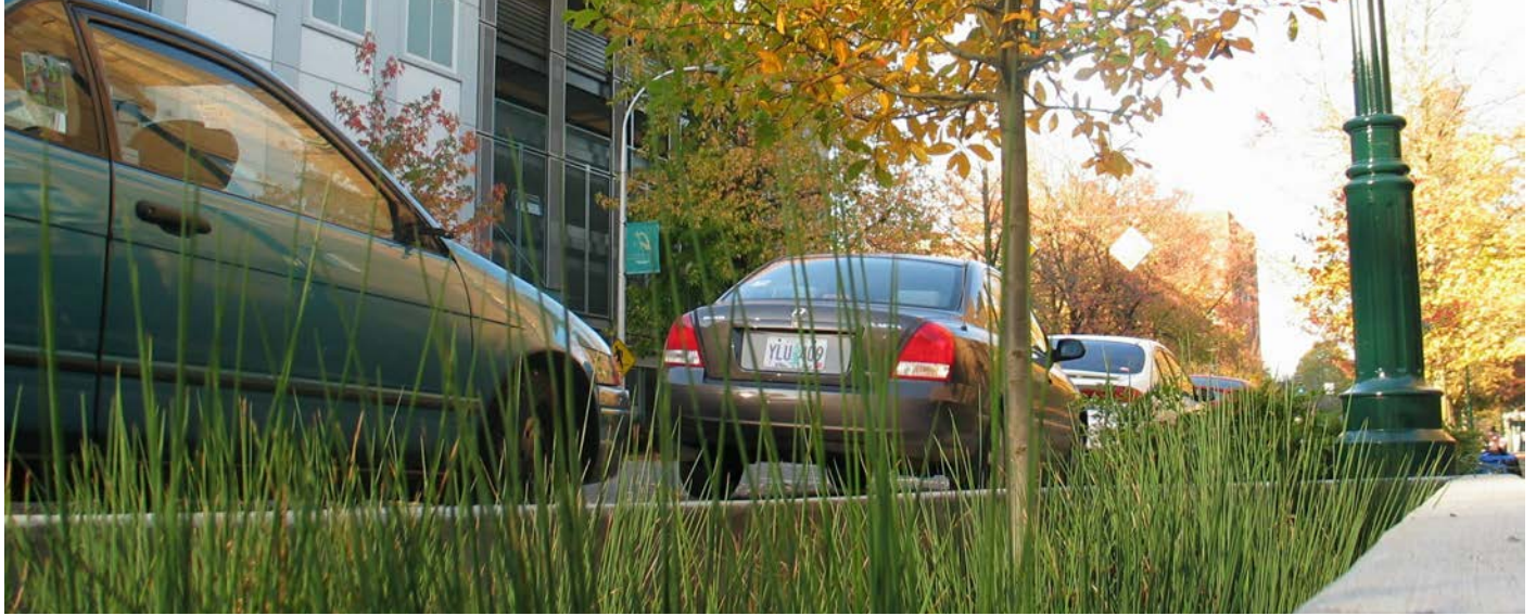
Bioretention planters assist with street greening and have stormwater management benefit.
